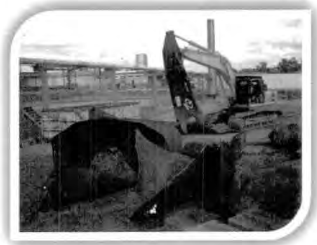
Figure 3.5.2 Managing dome steel for scrap recycling.
