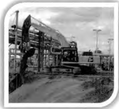
Figure 3.5.1 Removal of dome steel following insulation removal.
