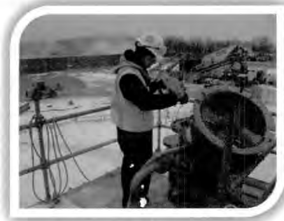
Figure 3.3.1 Manual grout level readings through open nozzle and air mover.
