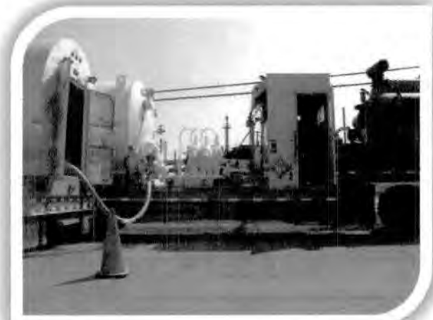
Figure 3.2.5 Nitrogen temperature control unit connected to rear of bulk liquid truck
